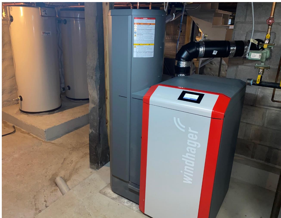
Figure 6 - a new pellet system installed in East Montpelier that replaced an old coal boiler.
